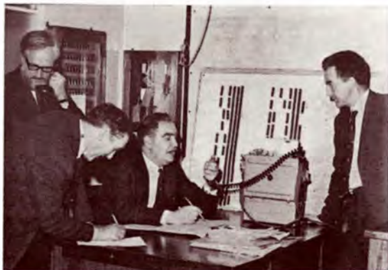
All systems go as Mr. G. Haughan ( District Engineer ) stands by, right, while load shedding instructions are broadcast over V.H.F. radio by Mr. A. Eyres ( systems engineer ) and over the telephone by Mr. J. Heaton ( production engineer ). Mr. J. M. Jones ( section engineer ) is kept very busy logging the details.
